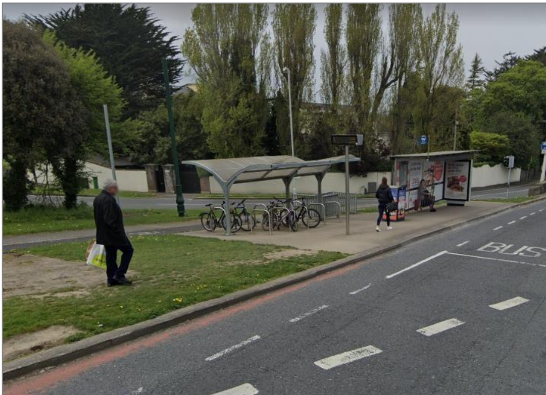
Figure 5.7 Covered Sheffield Bicycle Stands provided at a Bus Stop on the N11.
